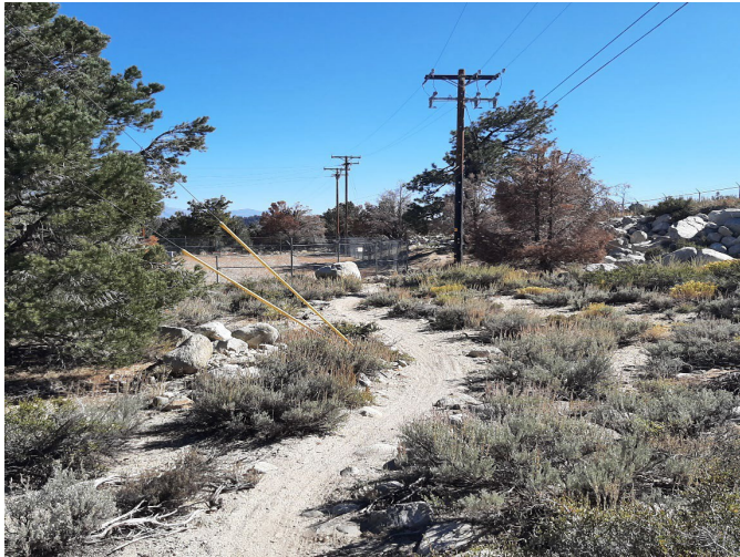
Looking east before SCE substation & FS sewer plant
