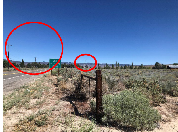
Figure 7: Existing overhead power lines looking north from the driveway.
