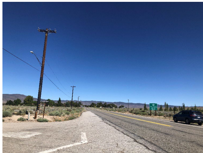
Figure 8: Existing overhead power lines looking northeast across from the driveway.
