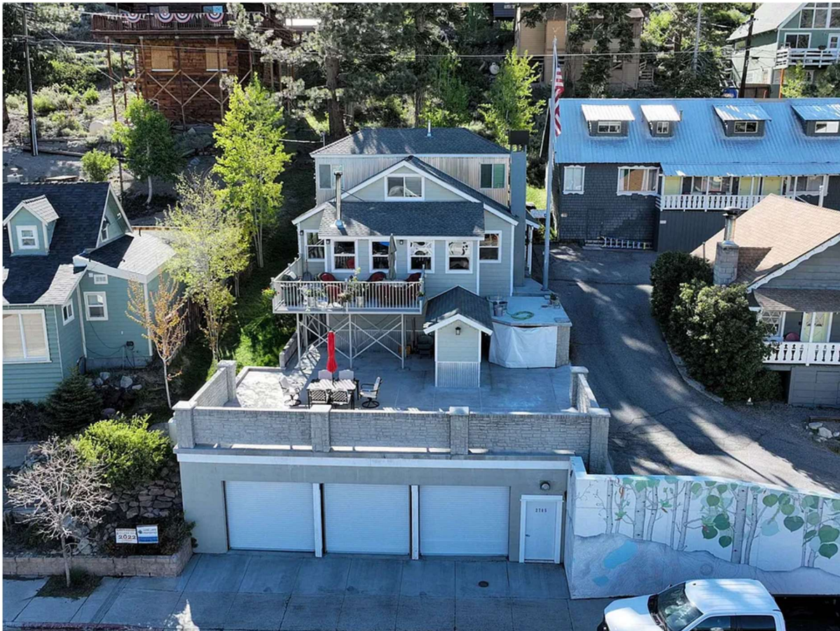
Figure 3: View of residence and garage from Highway 158.
