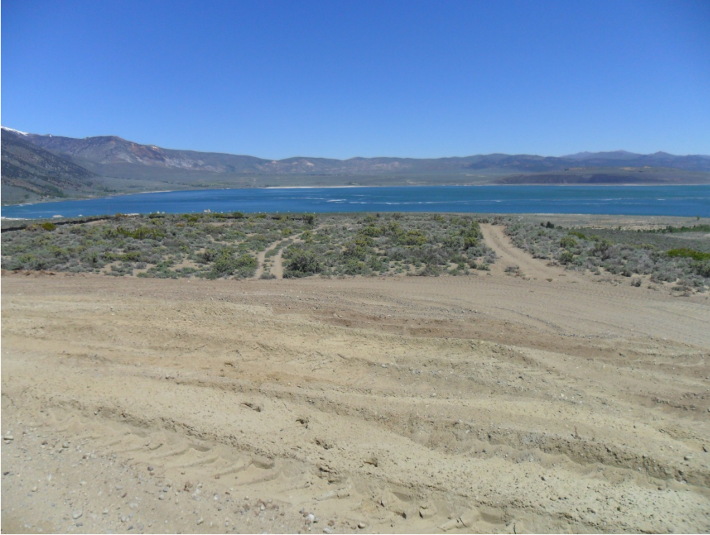
STOCKPILE CENTERLINE LOOKING NORTH
